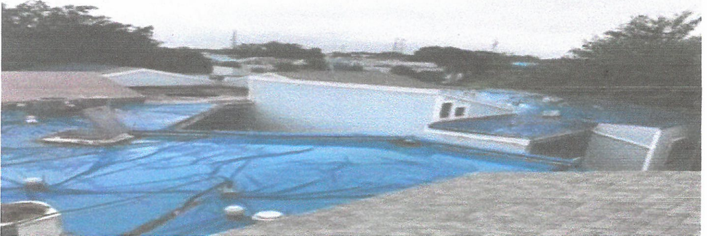
Fig 2 Shows roof overview
